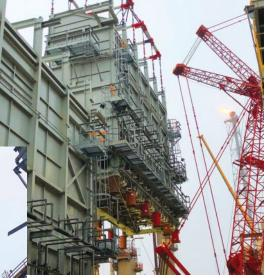
Successful 12-point super-lift ready for placement and fit up.
